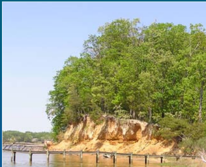
Sand bluff High bank subject to gravity, groundwater, wave attack forces
