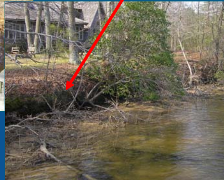
Eroding shoreline has scarp or undercut base
